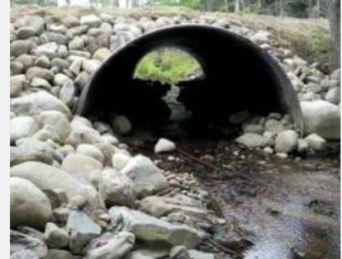
Replace undersized and perched culverts, remove clogs, armor inlets/outlets and install plunge pools
