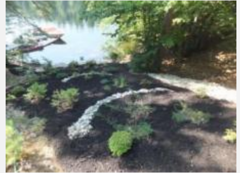
Erosion control mulch & vegetative planting
