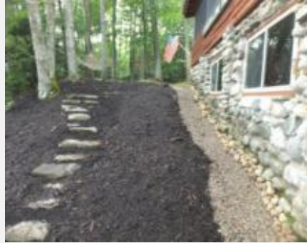
Dripline trench & erosion control mulch (Photo: AWWA)
