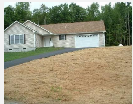
Install permanent BMPs once construction is complete including seed/ haying bare soil and installing vegetation on the shoreline (Photo: Maine DEP)
