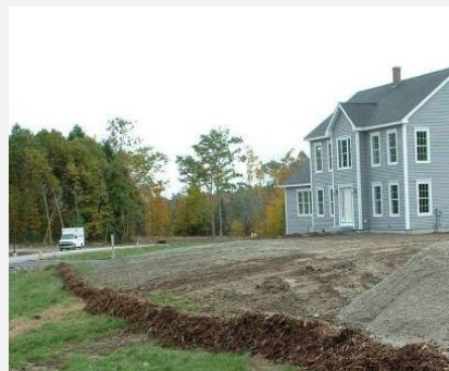
Install temporary BMPs such as an erosion control mulch berm prior to beginning construction (Photo: Maine DEP)
