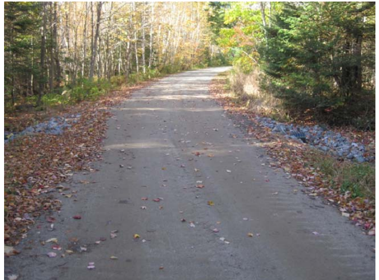
After: New, properly armored culvert and resurfaced, crowned road.
