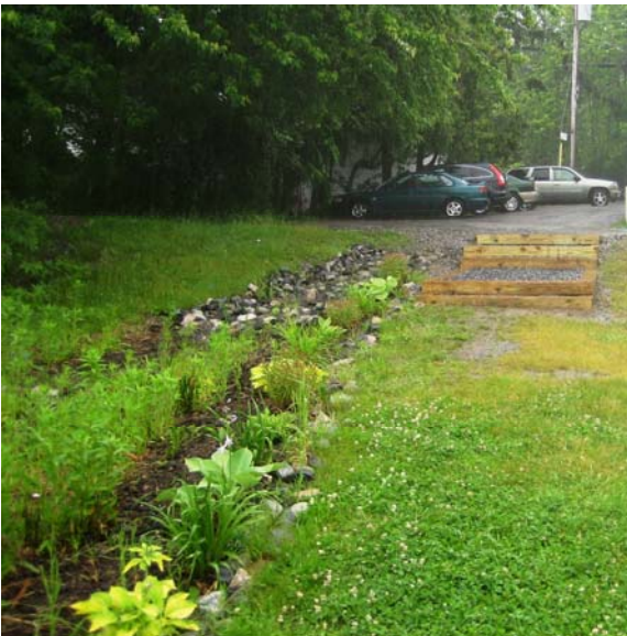
The rain garden and infiltration steps at Day's Store has had a lot of rain so we could see how it was working controlling the erosion caused by the run-off from Route 27.
