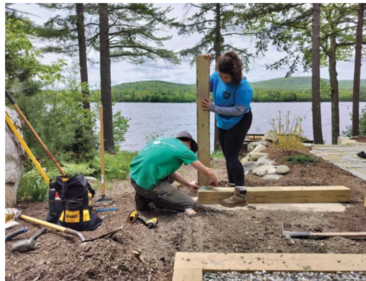
YCC crew members build an infiltration path.
