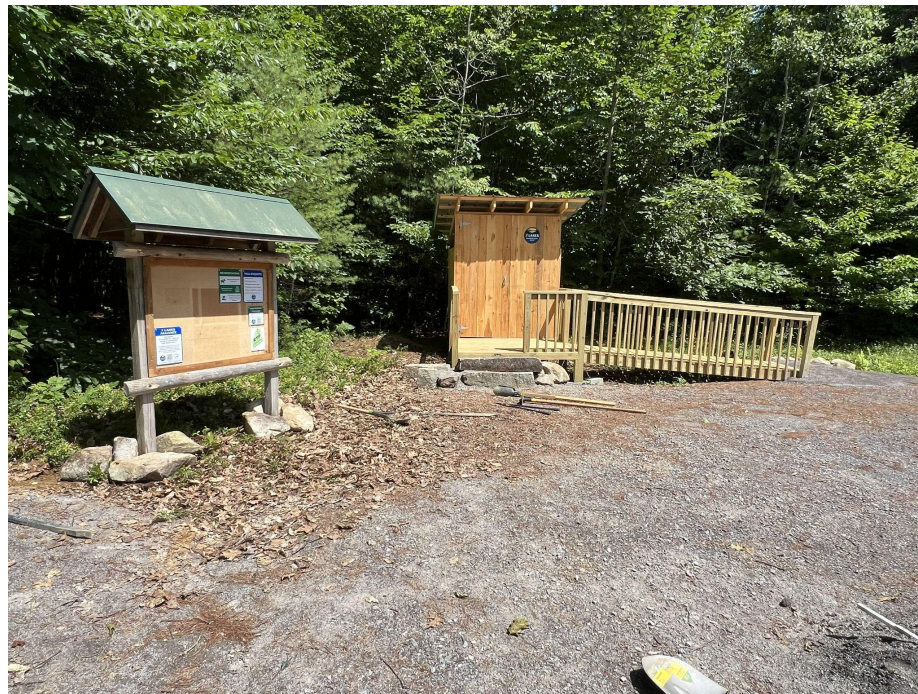
Homestead Trailhead: Wheelchair accessible composting privy
